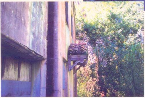
Photograph 2: DETAIL OF PARTIAL NORTH ELEVATION SHOWING HOOD OVER ENTRY DOOR WITH TILE ROOF.
