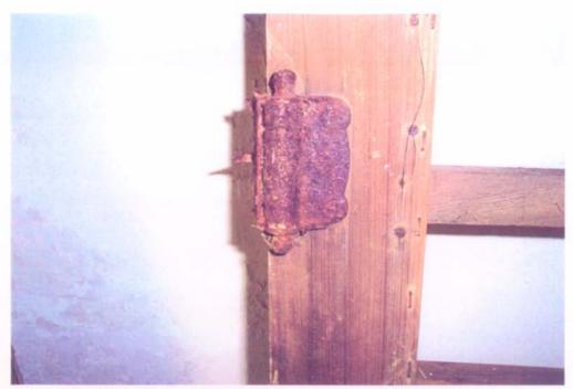
Photograph 17: DETAIL OF SELF CLOSING SCREEN DOOR HINGE.
