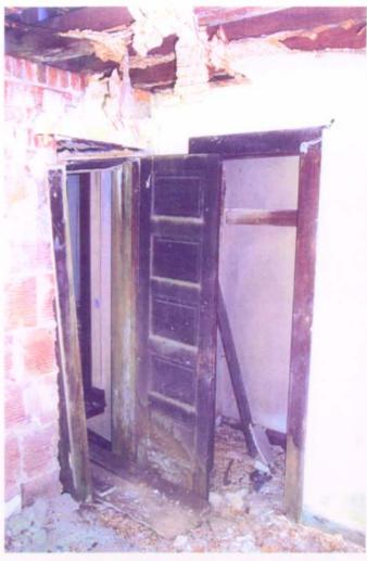
Photograph 11: INTERIOR ELEVATION OF DOOR AND CLOSET ON SECOND FLOOR SHOWING DETERIORATED CONDITION.
