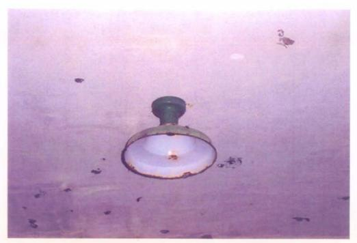
Photograph 21: DETAIL OF TYPICAL ORIGINAL GARAGE LIGHT FIXTURE.
