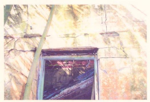
Photograph 4: DETAIL OF PARTIAL EAST ELEVATION WITH DOOR TO LAUNDRY SHOWING DETERIORATED STUCCO AND METAL LINTEL OVER DOOR.
