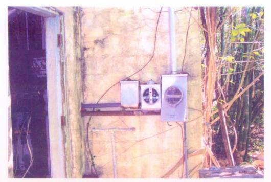
Photograph 5: DETAIL OF ELECTRICAL SERVICE ENTRY ON SOUTH ELEVATION.
